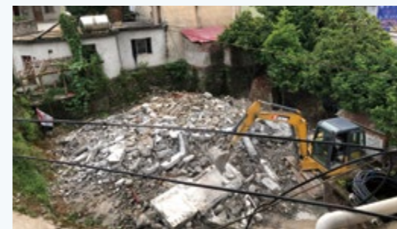
Health stations under construction in Jiangkou Village
