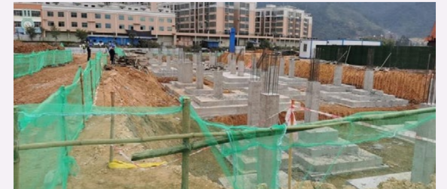
Construction of the Special School in Zhaoping County, Guangxi
