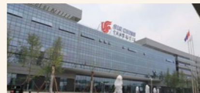
Air China Chengdu Tianfu Base
